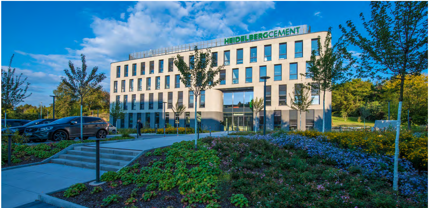
↑ HeidelbergCement Technology Center in Leimen
